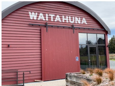
Beautifully restored old goods shed
